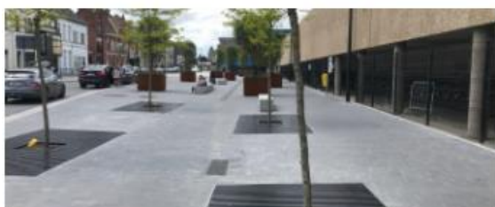
WAREGEM WAREGEM, R35 WESTERLAAN- NOORDERLAAN (2016.I.003)
